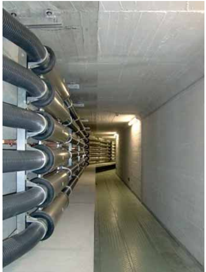
1350m of busbars have been installed
