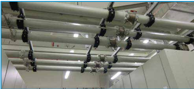
LINK® SF 6 insulated busbar system
