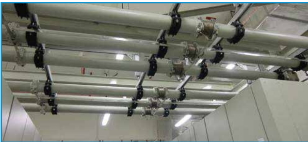
GASLINK® SF 6 insulatet busbar system
